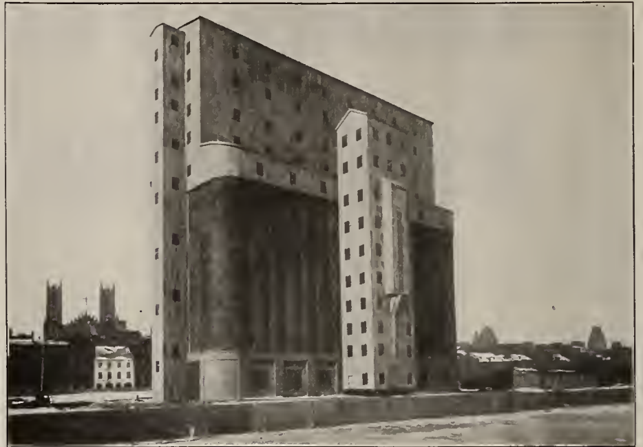
1,000,000-bushel fireproof Grain Elevator constructed of steel, for the Harbor Commissioners of Montreal, Canada.
